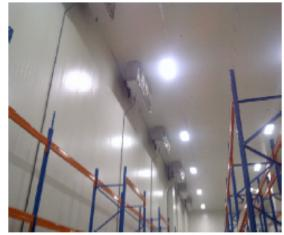
42m long x 12m high ceiling -22C Room, Blower (Evaporator) installation, anti-Freeze LED lamps with back up battery (optional), and heated drains.
