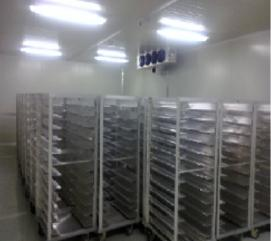
Chiller Room, Evaporator installation with ceiling suspension syster
